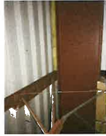
Gaps at Roof-Wall Intersection to be Sealed
