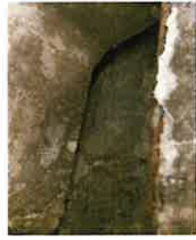
Gaps at Roof-Wall Intersection to be Sealed
