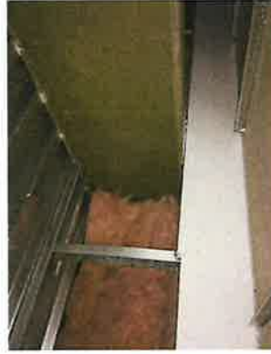
Interior View of Soffit to be Sealed
