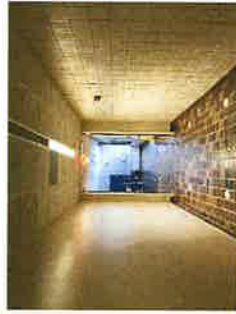
Dim Hallway Lighting
