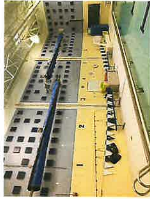
Existing High School Pool Cover
